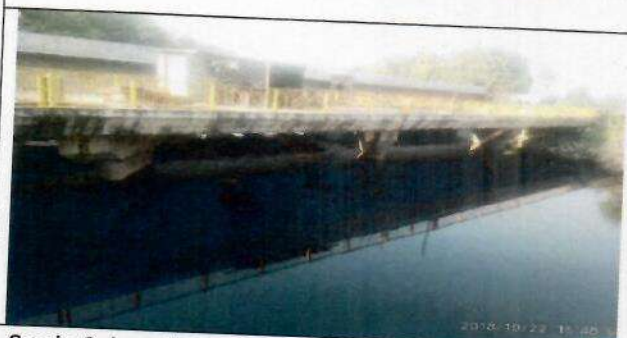
Sarda Sahayak canal at Umaria Bridge (22.10.2018)
