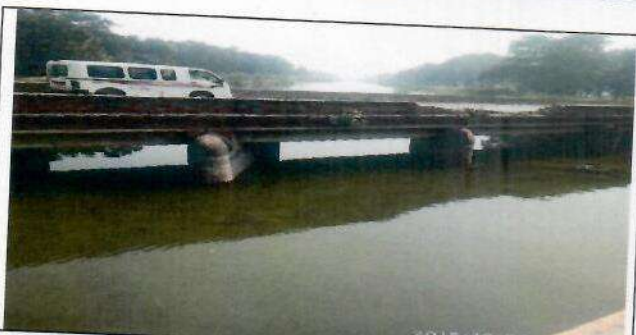
Sarda Sahayak canal at Umaria Bridge (23.10.2018)
