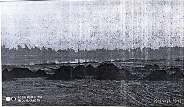
P11: Katcha Lagoon under dismantling Process
