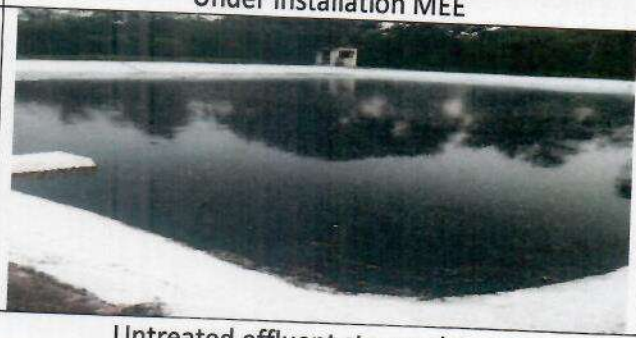
Untreated effluent storage lagoon
