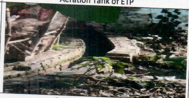
Outlet of bypass drain
