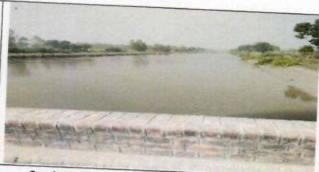
Sarda Sahayak canal at Umaria kala Bridge (23.10.2018)
