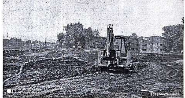
P14: JCB in Bio-compost Yard
