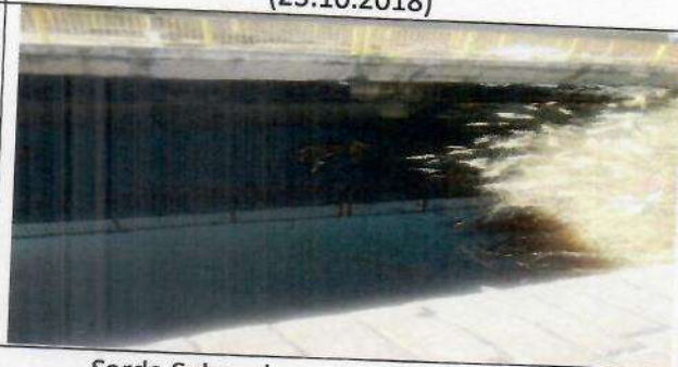
Sarda Sahayak canal at Umaria Bridge (22.10.2018)
